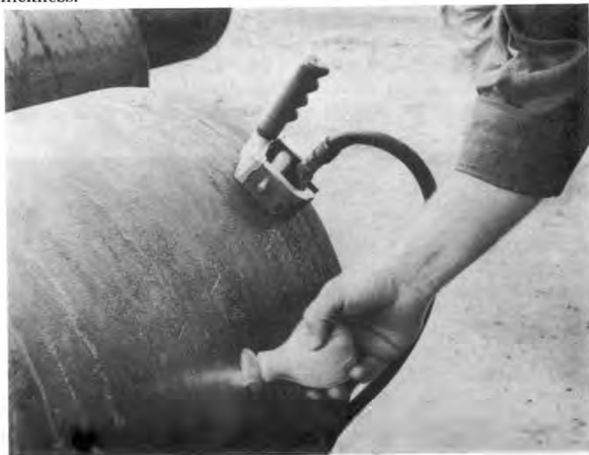
Fig. 214—Close-up of Inspection of 24 Inch Line Pipe, Three-Mile Mississippi River Crossing.
