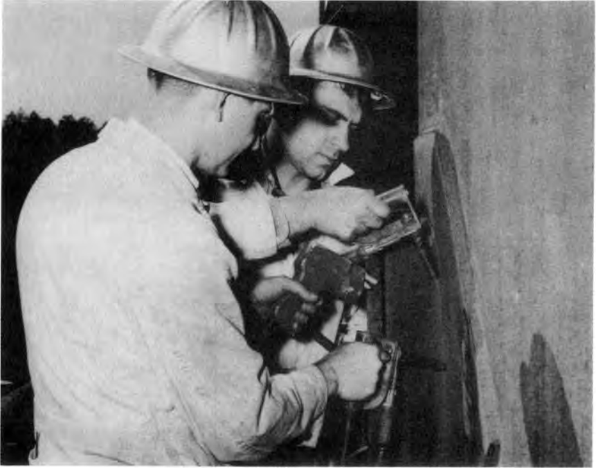
Fig. 224—Testing a Welded Oil Storage Tank.
